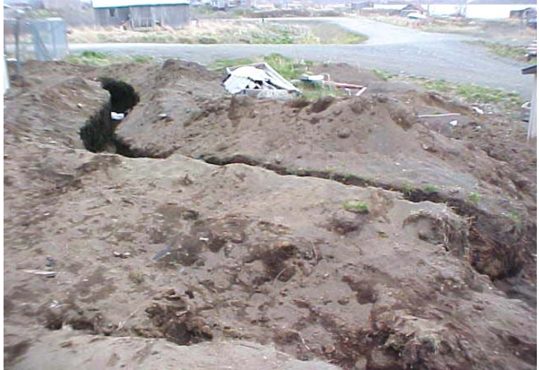
Figure 4. View of southeast portion of the sewer line trench, view northwest.
