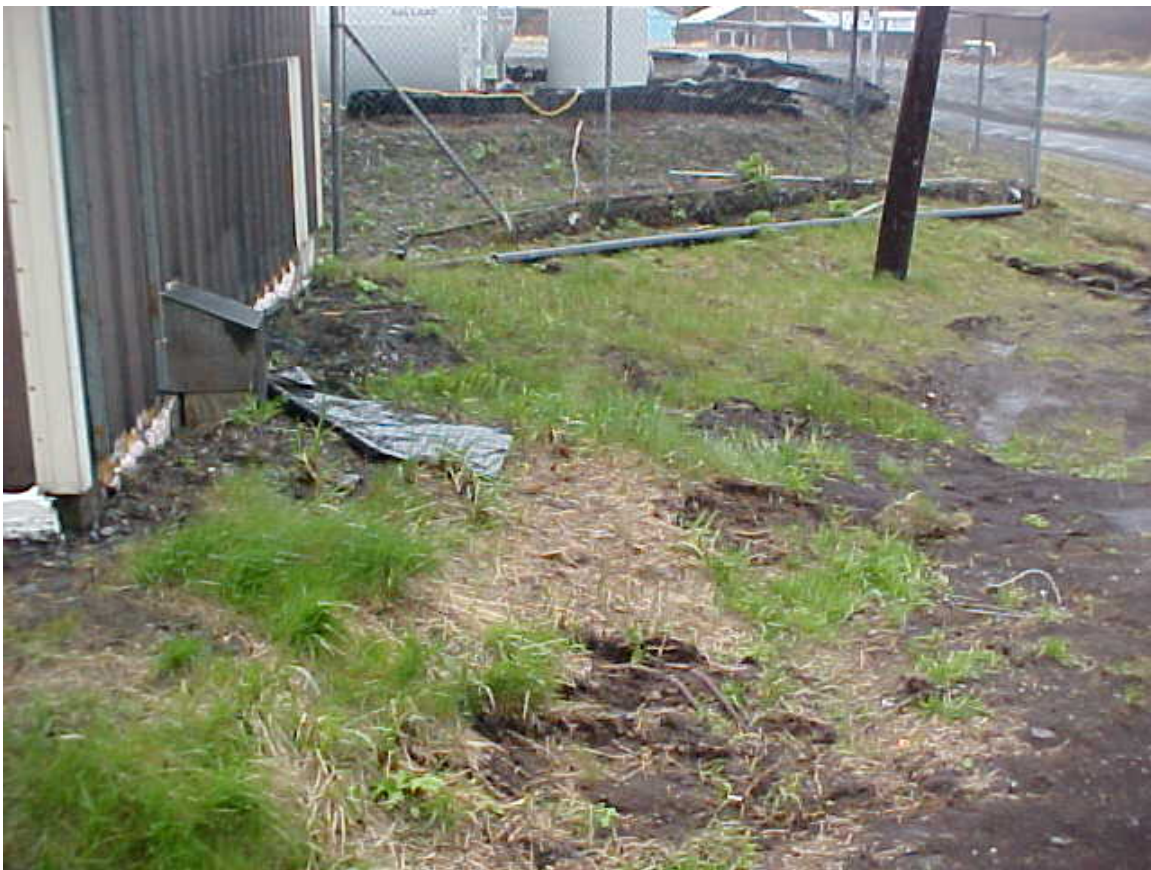
Figure 12. Location of generator building extension. Building will be extended to location of existing utility pole.
